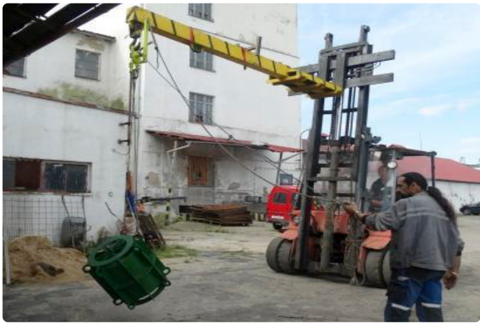
• Transportation to the test area
